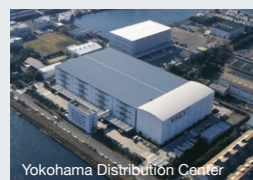
Yokohama Distribution Center
